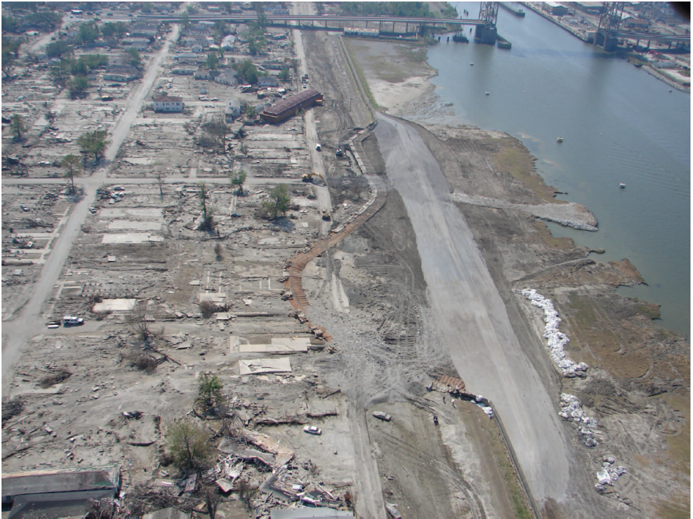
Fig. 9. (Color) Oblique view of the (south) levee breach at the Inner Harbor Navigation Canal into the lower Ninth Ward
