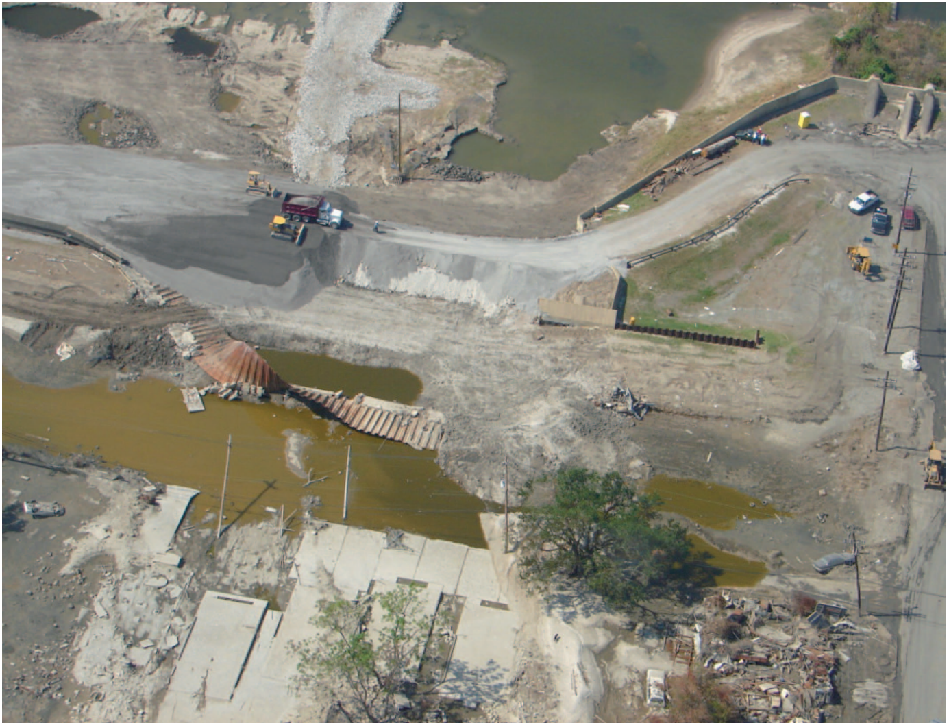
Fig. 5. (Color) Aerial view of the north breach on the east bank of the IHNC, at the west end of the Lower Ninth Ward
