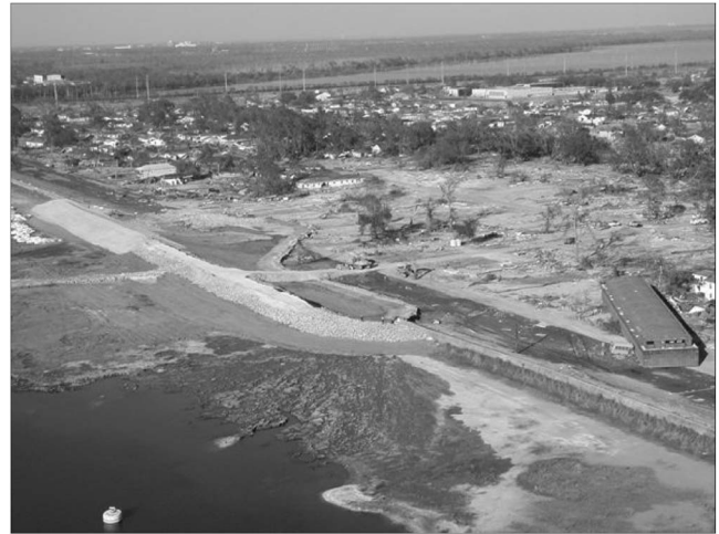
Fig. 17. Reverse crevasse splay produced by reverse drainage out through the foundation soils beneath the interim repair embankment section; south breach IHNC at the Lower Ninth Ward (IPET 2006)
